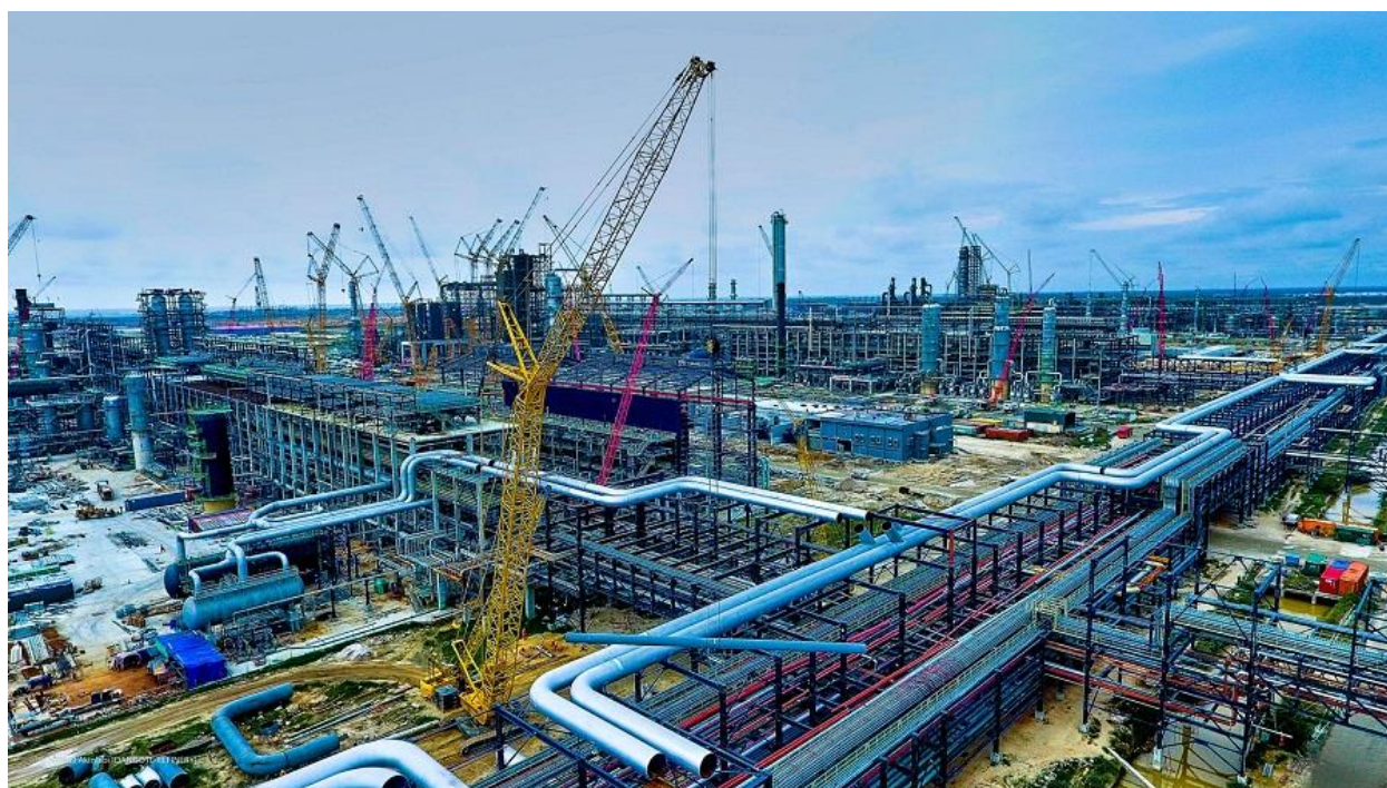
Figure 2. The Dangote Refinery in Lekki Free Trade Zone, Lagos, Nigeria (Ubah, 2022)
