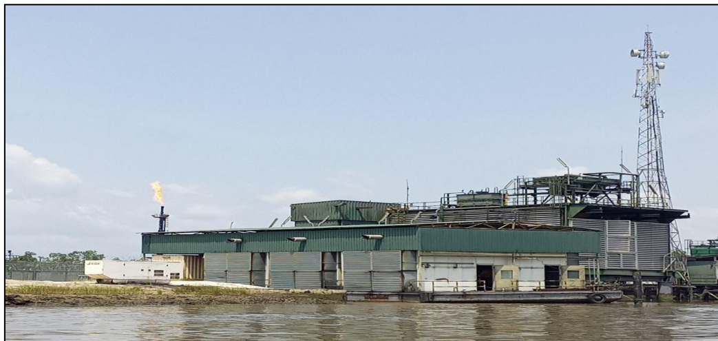
Figure 2: Picture of an actual flaring site in Delta State.
